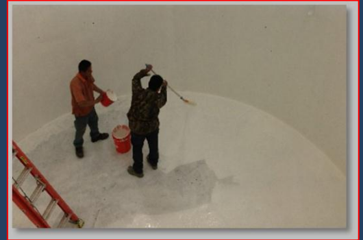
TANK LINING USING MCCRORY 500
